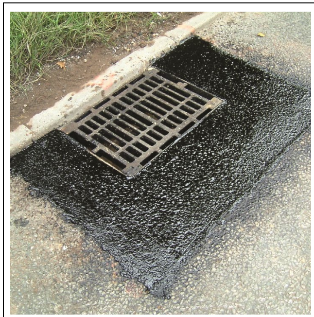
Figure 4 Surface reinstated with Ironmaster Patch
