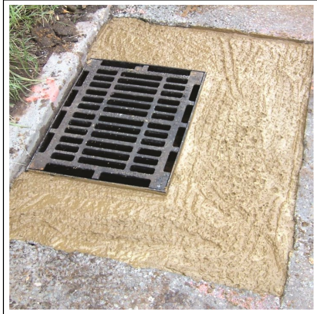
Figure 3 Ironmaster Infill applied
