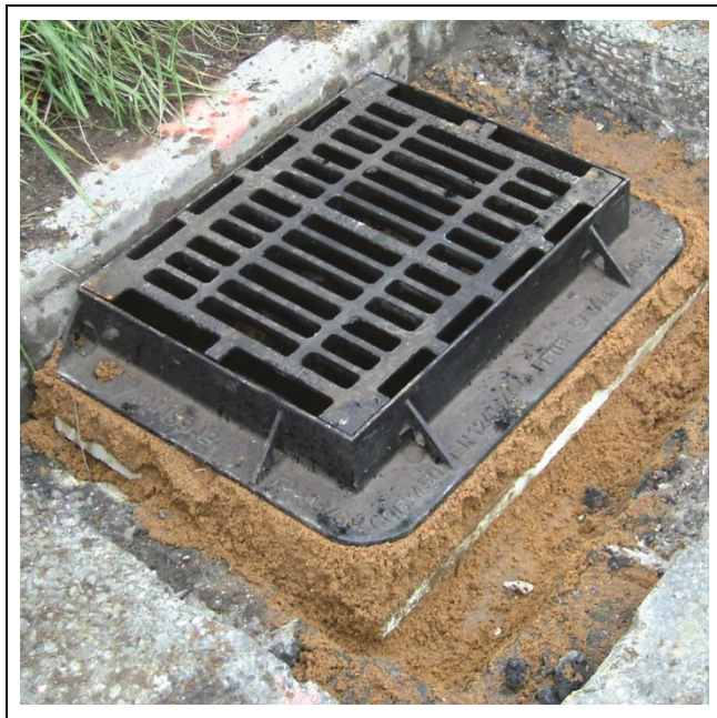
Figure 2 Frame bedded on Ironmaster Mortar P
