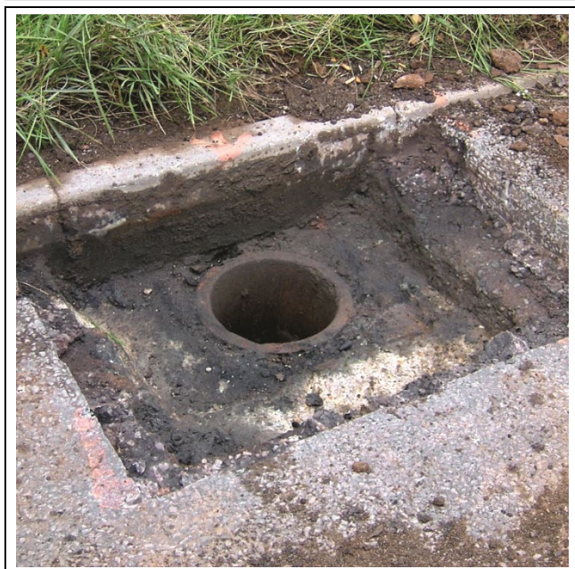
Figure 1 Prepared excavation
