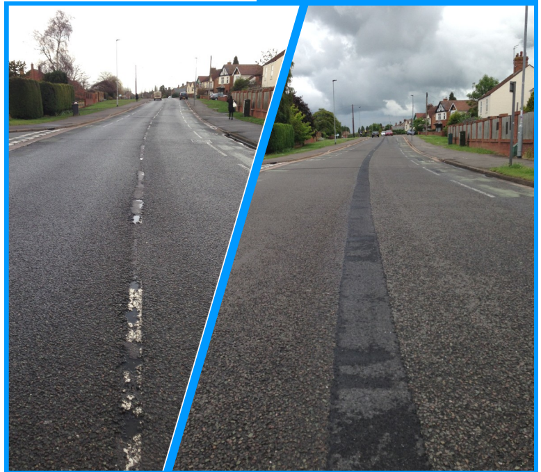
Transverse & Longitudinal repairs
