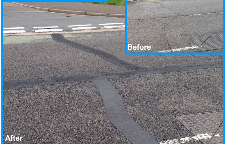
Transverse & Longitudinal repairs
